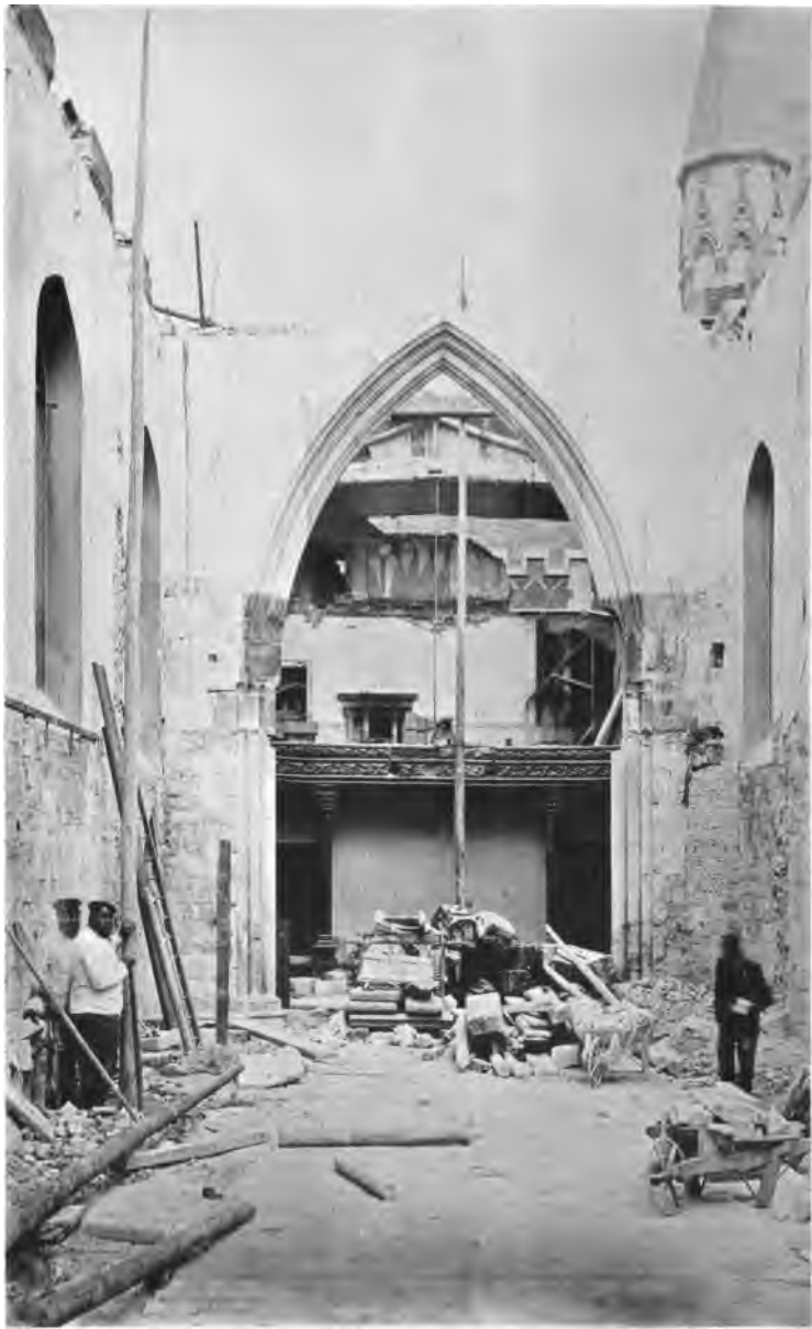
QUIRE ARCH. LOOKING WEST.
